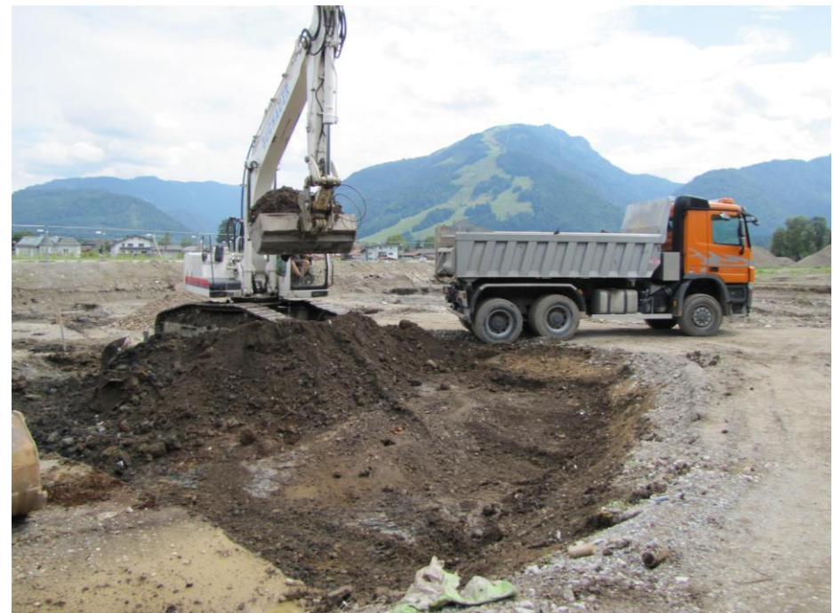
Abb. 14: Interner Materialtransport (7. August 2014)
